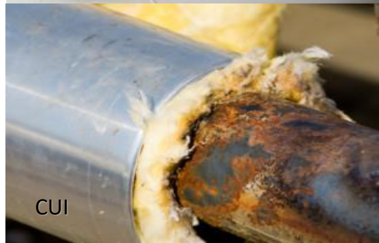
Coating and wrapping
